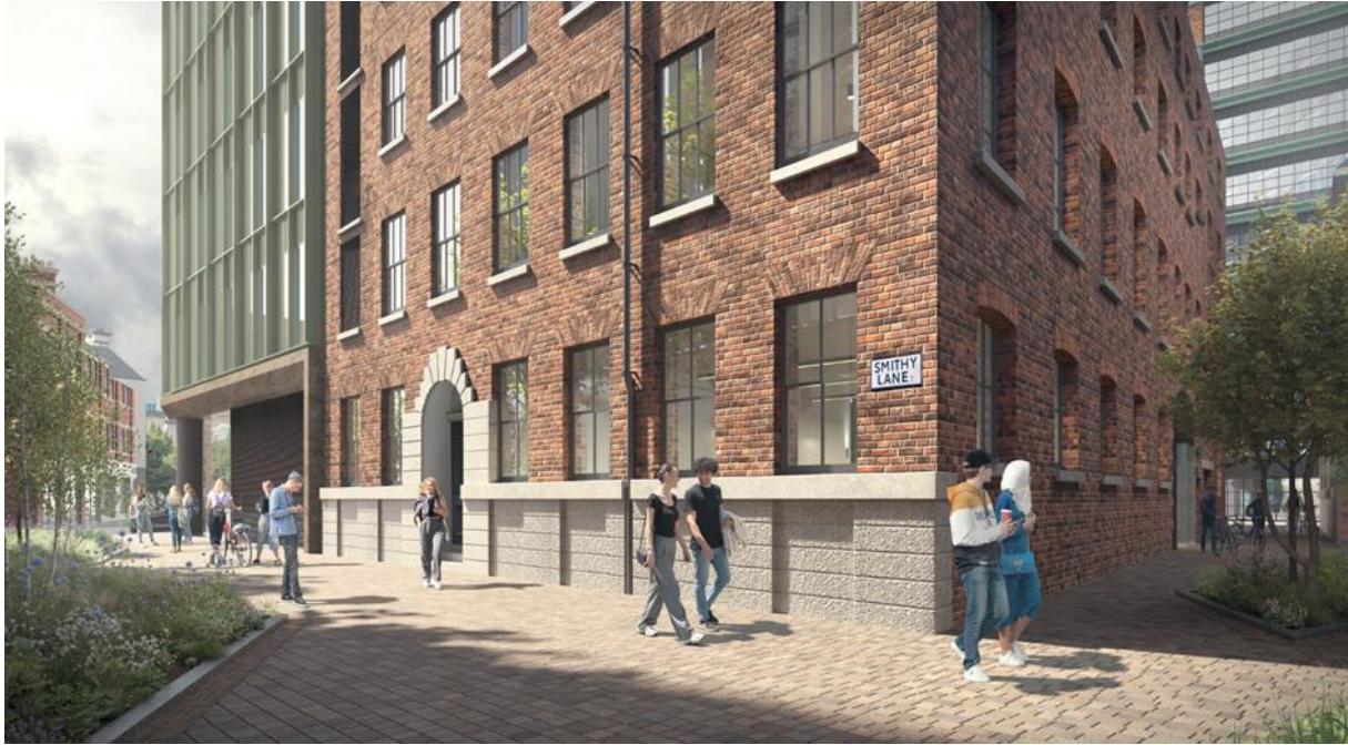
Image b) The refurbished Warehouse at 3 Smithy Lane
